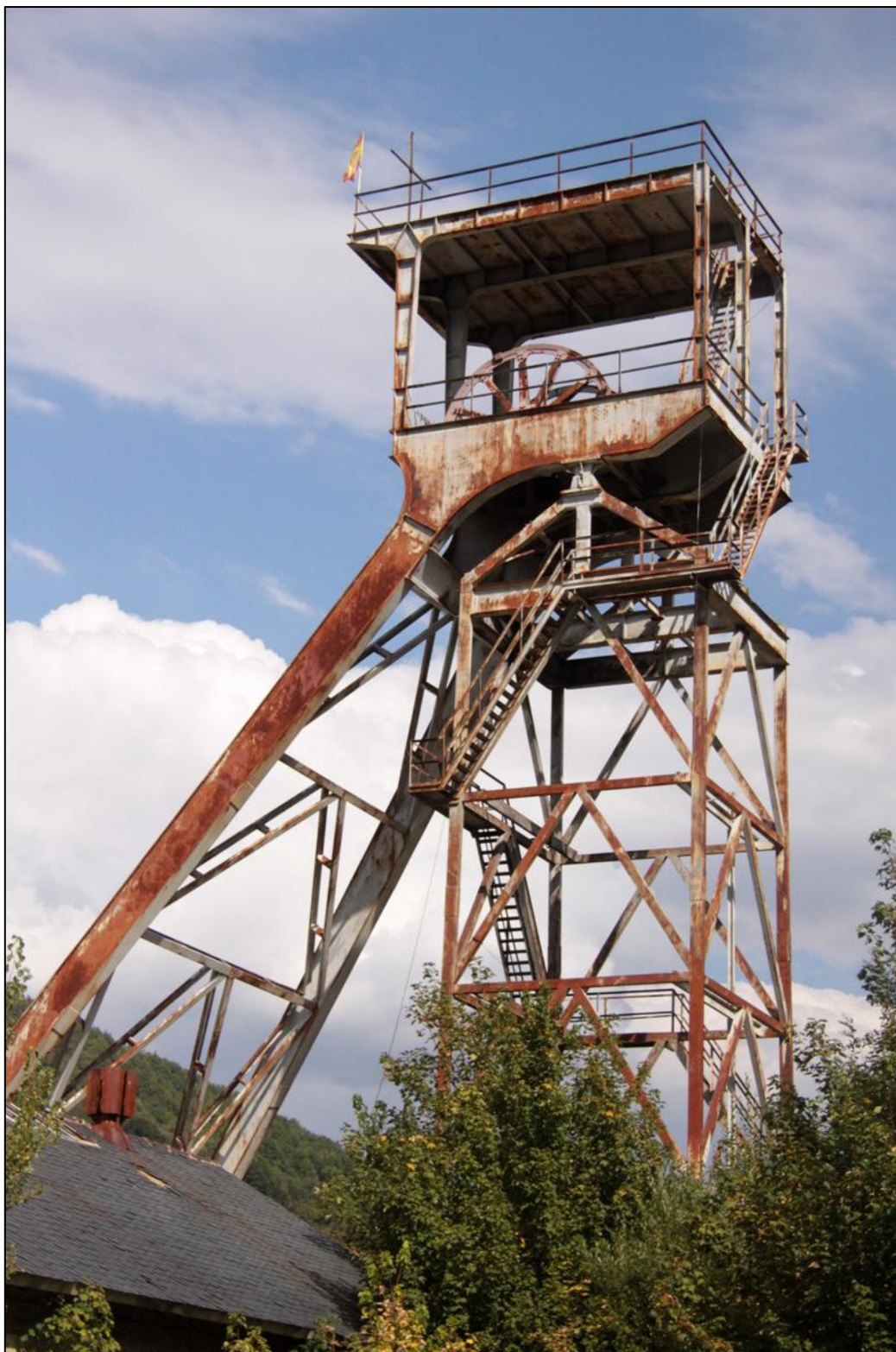
Figura 22: Pozo María , Villablino, León (Fot.: J.M. Sanchis, 2013)
